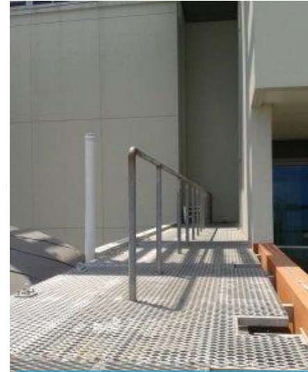
RAILING AND CATWALK
